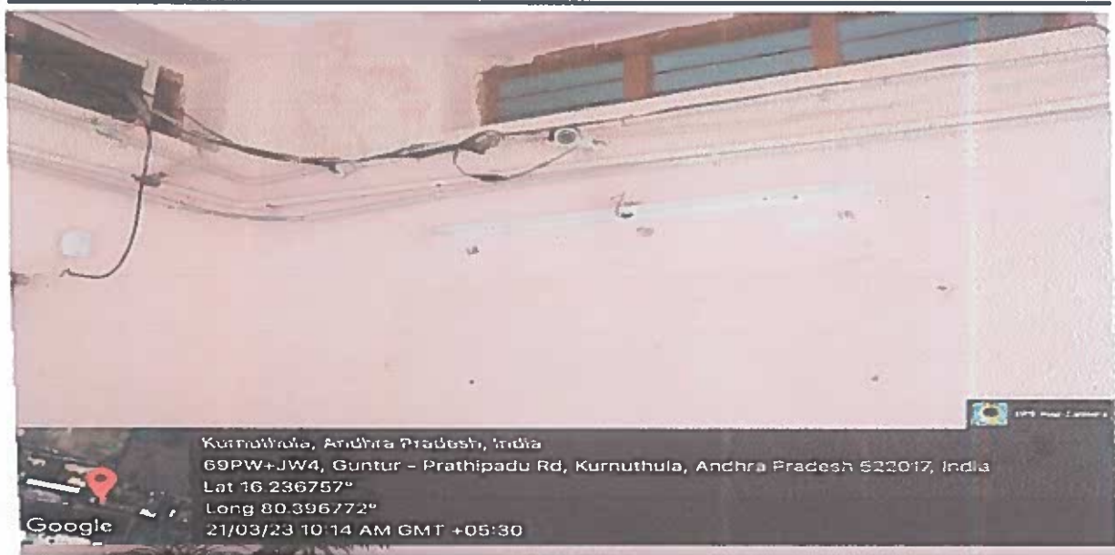
ADMIN BLOCK CC SERVIVELANCE
